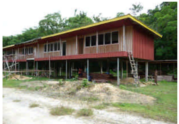
Kokeqolo High School (Munda). A new building in which SMCS helped pay for the roof.
